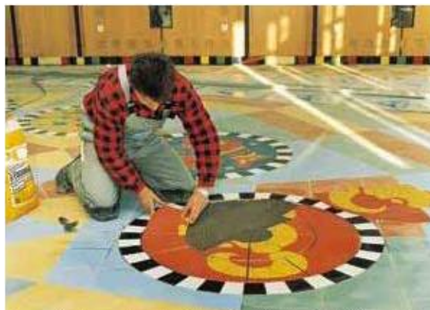
Secure laying of tiles with Mastertile FLX 23
